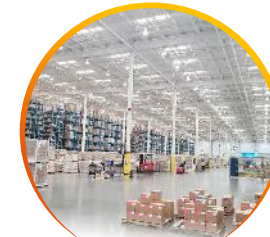
Nashville facility now fully operational
